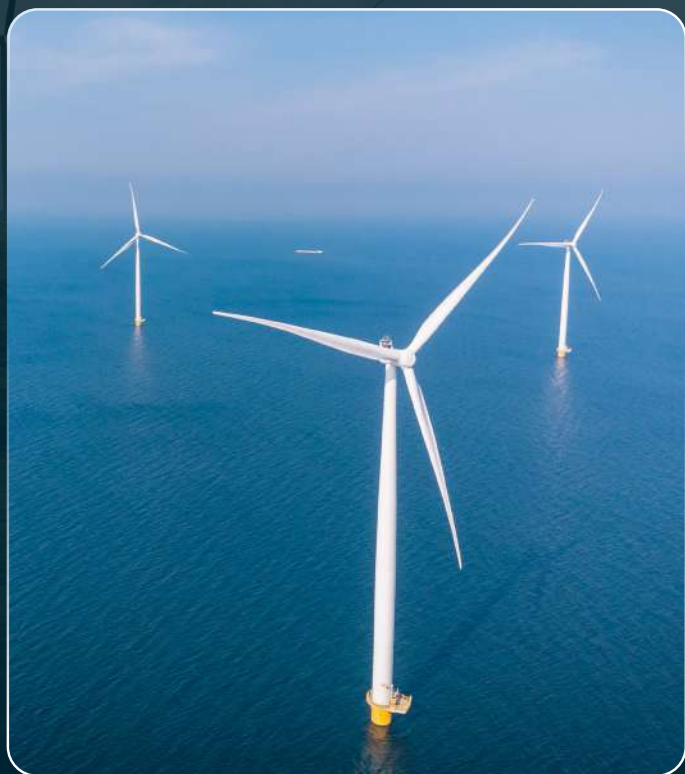
Offshore Wind Farm
