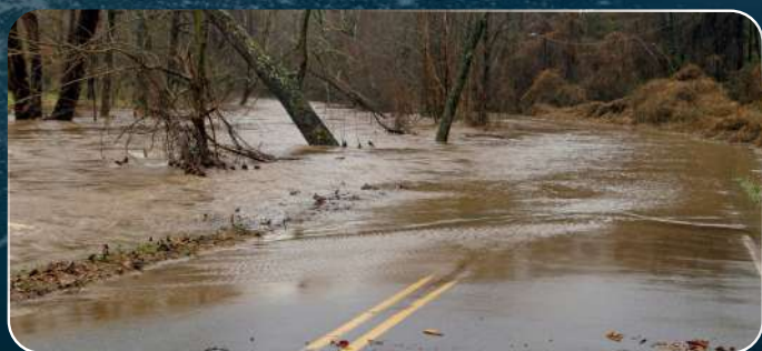
Flooding caused by heavy rains
